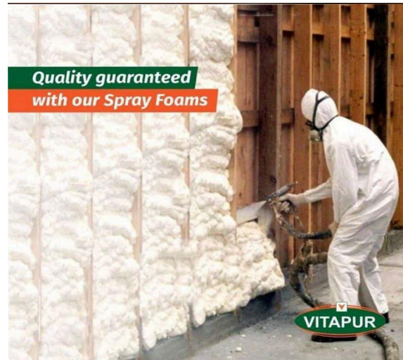
Spray foam Application
